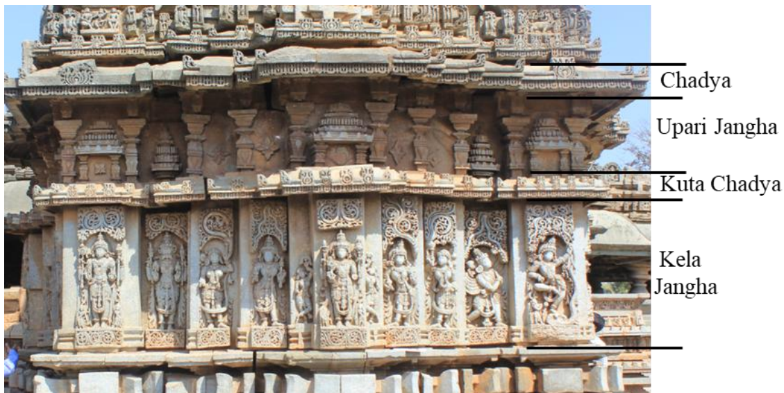
Figure 4: Wall detail of Hoysala Temple.
