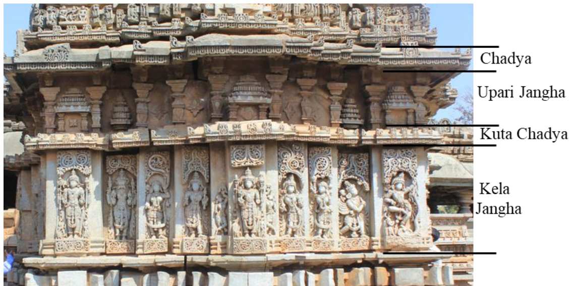
Figure 4: Wall detail of Hoysala Temple.
